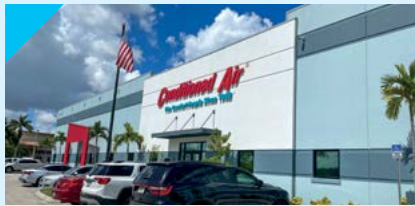
CONDITIONED AIR Fort Myers, FL
